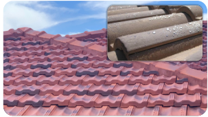
Roof Tiles Restored
