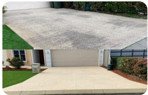
Exposed Aggregate Restored
