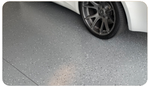
Garage Epoxy Flooring
